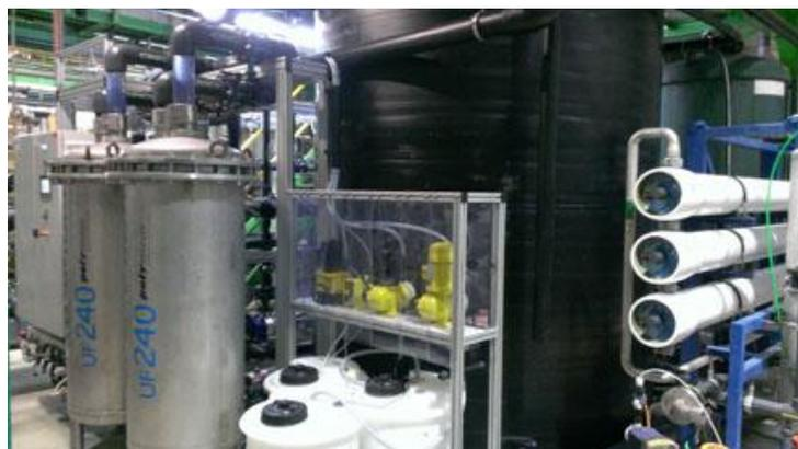
The picture shows a water treatment plant with three pressure pipes for reverse osmosis membrane elements (right) and two ultrafiltration (UF) modules of the type Gigamem UF 240 (left). The technologies complement each other perfectly, as around a third of all newly built reverse osmosis systems have upstream ultrafiltration. Photo: Polymem SA
